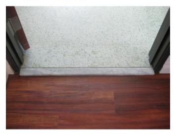
Bathroom entrance: The elevation of the bathroom floor and the hallway floor are not in compliance with ADA regulations.
