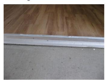
Patio Door: The difference of elevation between the dining room floor and the patio area is 1 3/4". The ADA regulation states that the fall between the two elevations is 1/4" per foot. Not in ADA compliance.
